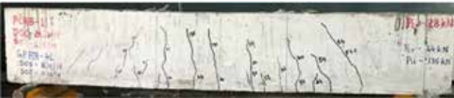
Fig 11. Crack pattern in beam retrofitted with 4 layers of glass FRCM
