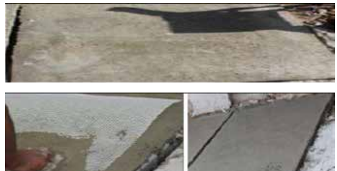
Fig. 4. Strengthening of slabs with glass FRCM
