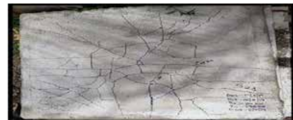
Fig. 10. Crack pattern of slab-S21 and S22
