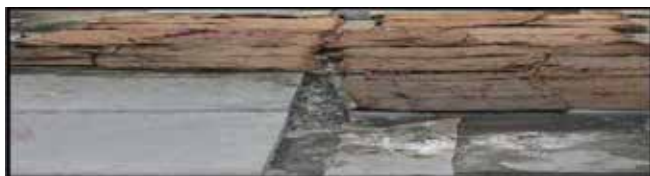
Fig 3. Curing of slabs
