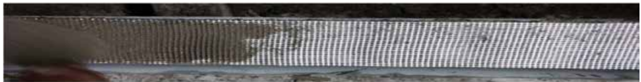
Placing glass fabric and mortar impregnation
