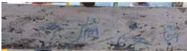
Figure 9 Crack pattern in CB-2
