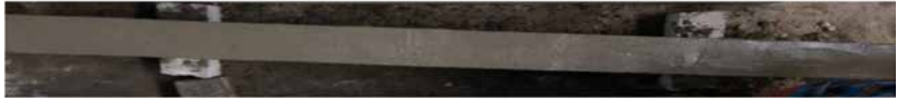
Placing of mortar on the prepared surface
